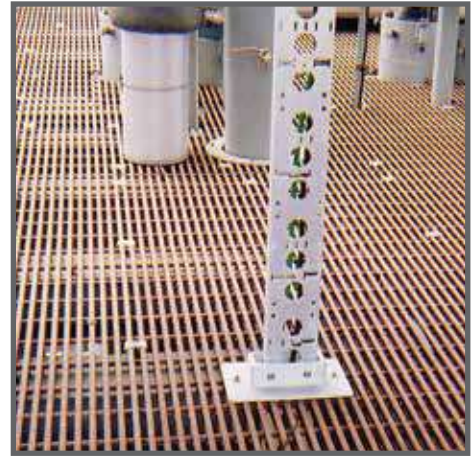
Offshore Oil & Gas Platform
