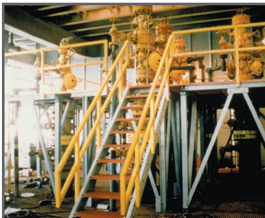
Dynaform support structure and square tube railing provide a high level of corrosion resistance for this offshore platform.
