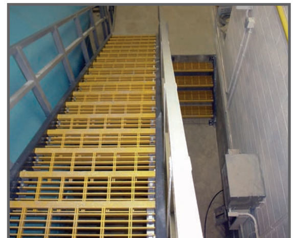
The stairway above utilizes Fibertred moulded stair treads to provide tank access at a pumping station.
